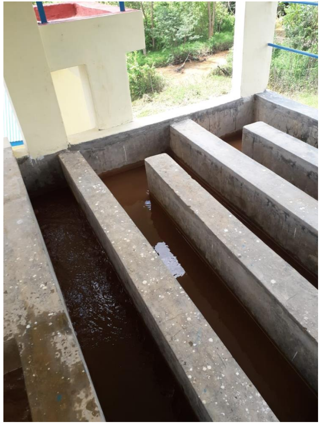
Raw Water Chambers, Baffles, Solution Tanks and Rehabilitated CFU
