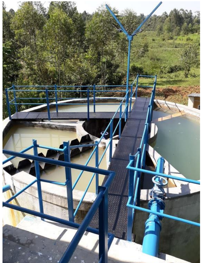
Raw Water Chambers, Baffles, Solution Tanks and Rehabilitated CFU
