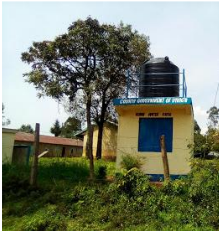
Top: Newly Constructed Water Kiosk with roof slab and Storage Tank
