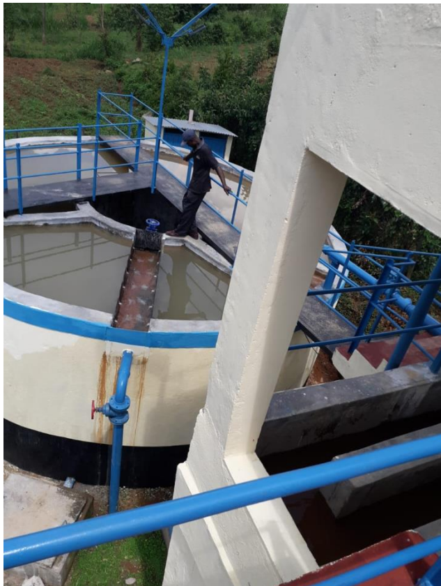
Raw Water Chambers, Baffles, Solution Tanks and Rehabilitated CFU
