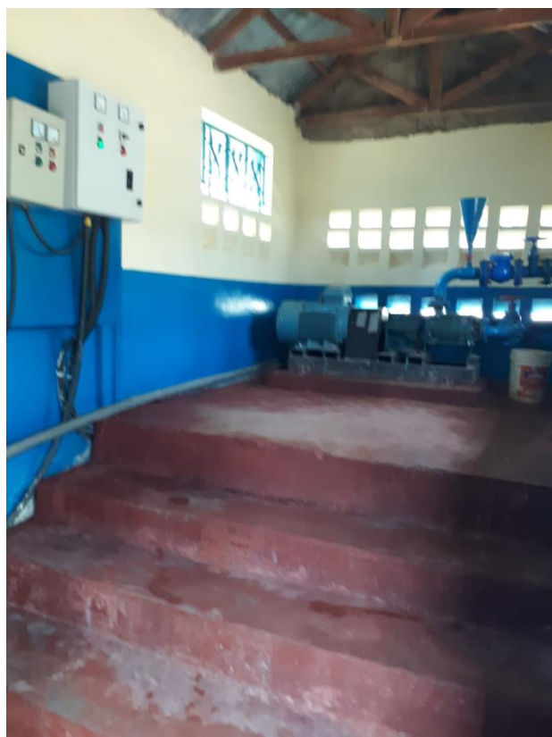
Rehabilitated pump house, High Lift, Low Lift and control panels
