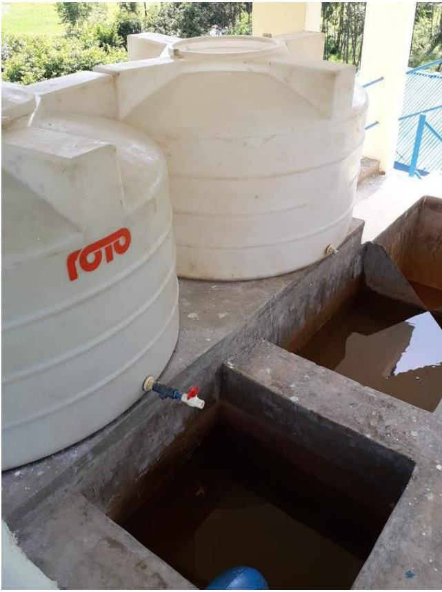
Raw Water Chambers, Baffles, Solution Tanks and Rehabilitated CFU
