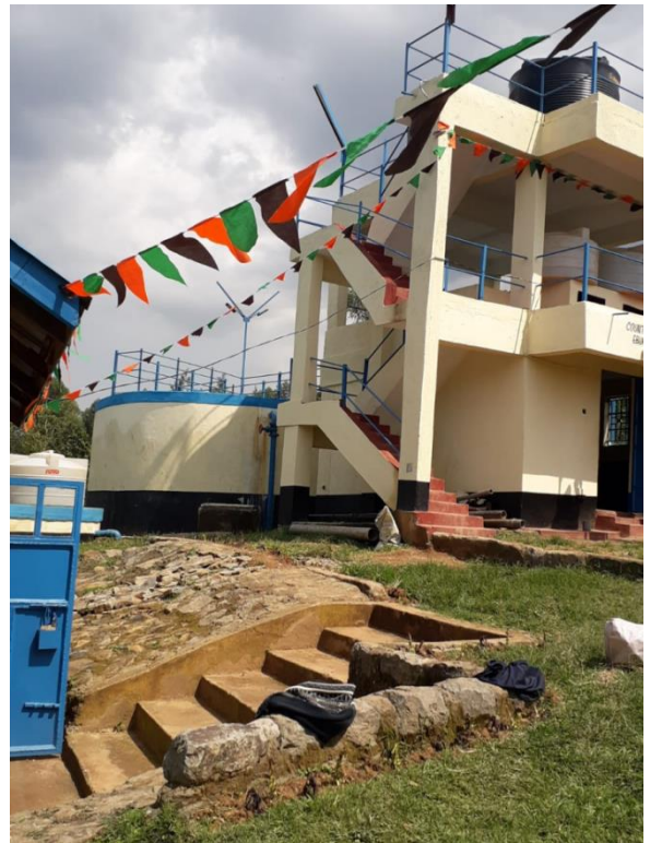
Treatment plant with backwash tanks and chemical store
