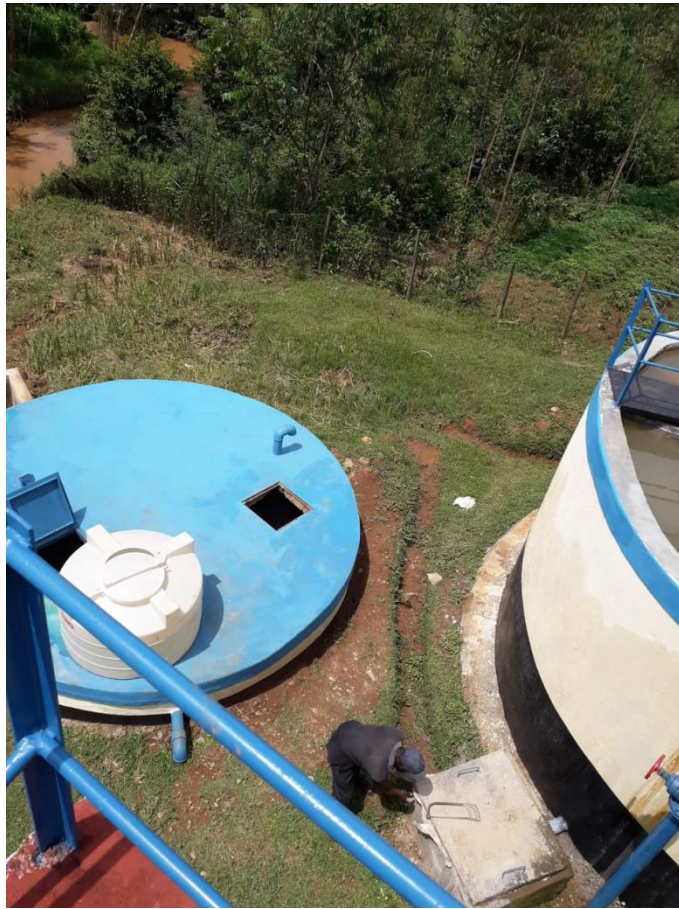
Rehabilitated clear Water Sump, gate and one of the sign posts
